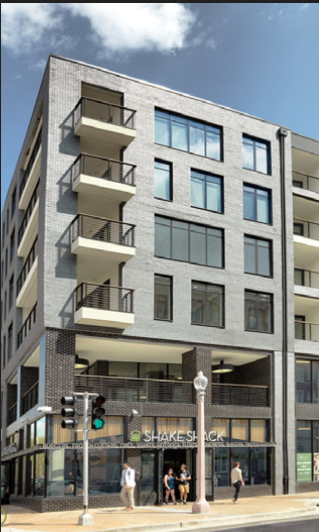
40 N. EUCLID 24 Gauge 4" Round Downspout, Custom Collector Boxes
