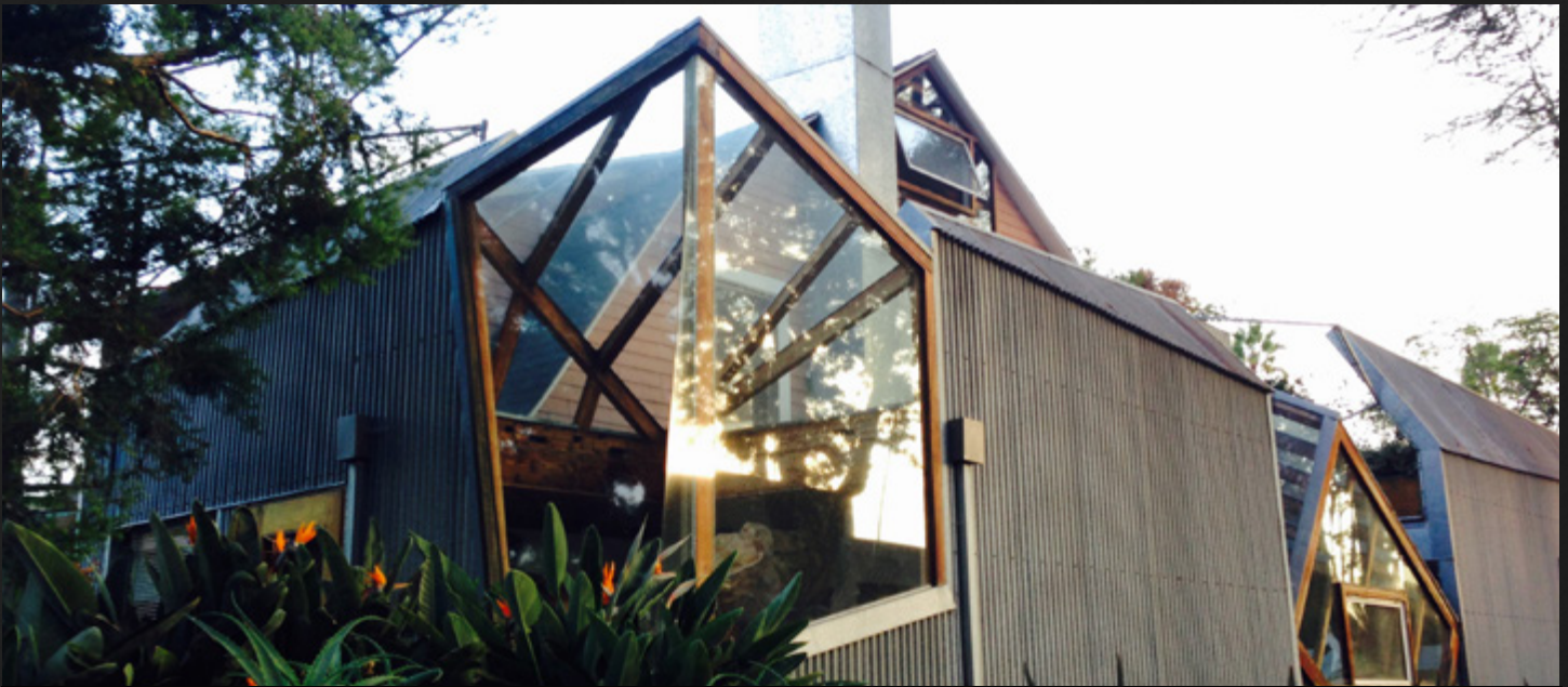
FRANK GEHRY RESIDENCE 24 Gauge 304 Stainless Custom Collector Head, 24 Gauge 304 Stainless 3" Round Downspout & Custom Elbows
